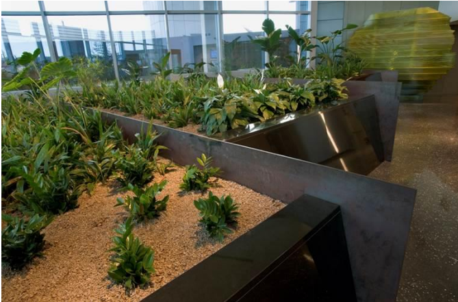
Constructed Wetlands Treatment Unit
