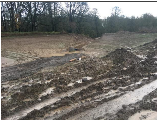
North stormwater pond under construction. Sediment fence was in good condition.
