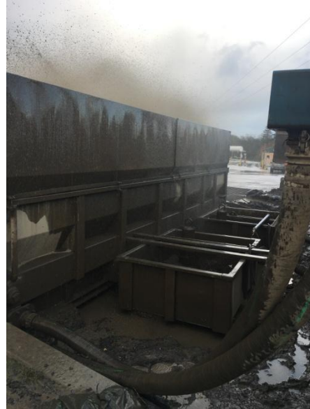
Muddy water at wheel wash. Landfill manager stated that this problem is caused by water/sediment reservoirs that are too small and pumps that are too powerful, and therefore stir up sediment in reservoirs. They are working on replacing this wheel wash. A date for replacement has not been determined.
