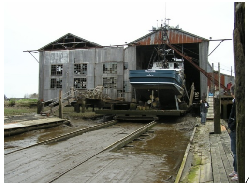
2012 photograph that shows a fishing vessel pulled into one of AMCCO's shipways.
