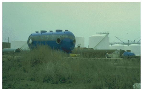
Above ground storage tanks
