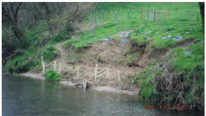
Livestock exclusion and bank stabilization project in the lower Big Elk Creek watershed (Photo courtesy Lincoln Soil and Water Conservation District)
