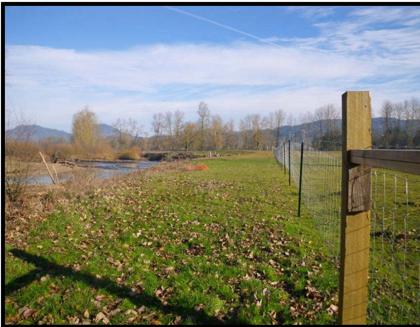
Post site preparation and fence installation. Pre riparian planting. January 2012
