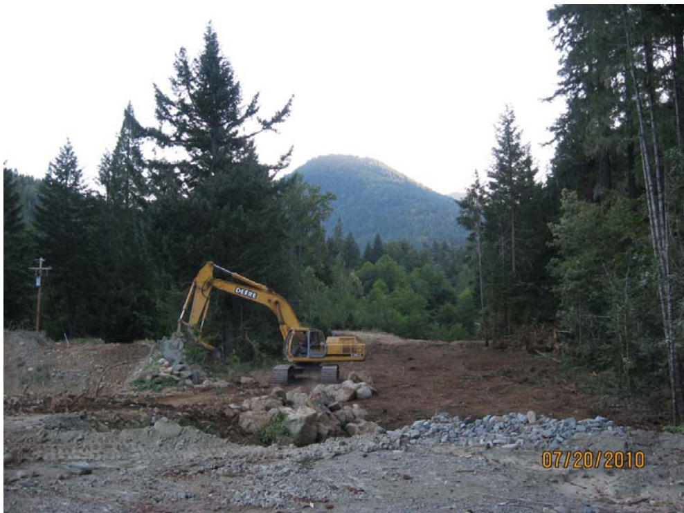
Post-Project Phase II Reach On Private And Public Land. Downstream View Of A Portion Of The Phase II Project Restoration Work Completed In 2010. Note Excavation Depths Were Approximately 20 Feet.
