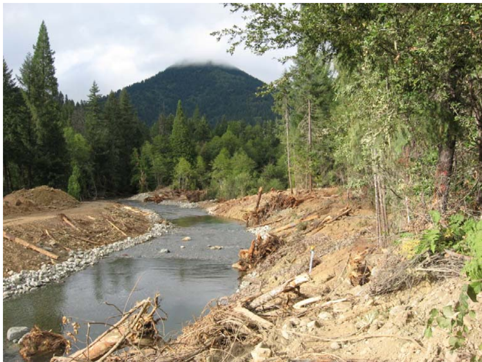
Post-Project Phase II Reach On Private And Public Land. Downstream View Of A Portion Of The Phase II Project Restoration Work Completed In 2010. Note Excavation Depths Were Approximately 20 Feet.
