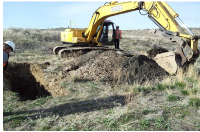
Test pit exploration to find horizontal landfill extents.
