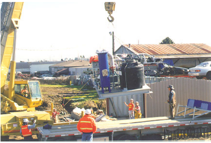
Installation of new landfill gas control components.
