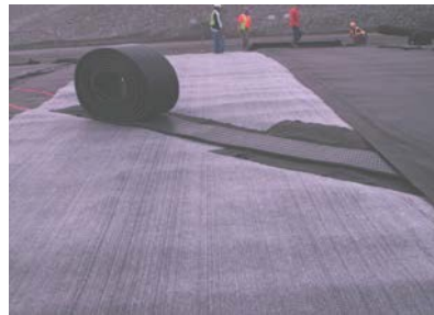
Landfill cap improvements.
