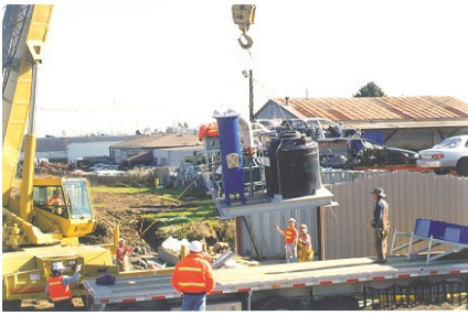
Installation of new landfill gas control components.
