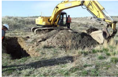
Test pit exploration to find horizontal landfill extents.
