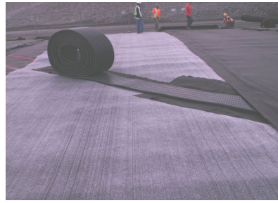
Landfill cap improvements.
