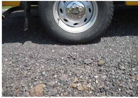
Compacted Grindings on Road Shoulder
