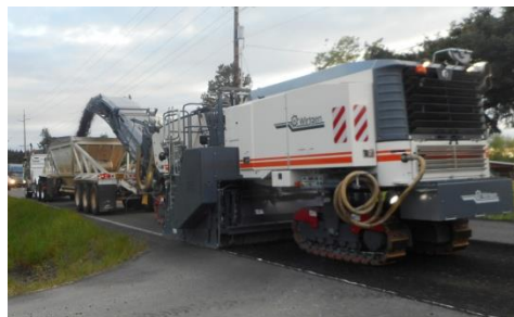
Asphalt Grinding Equipment
