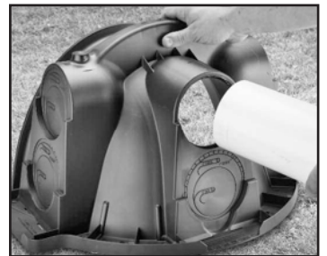
5. Insert inlet pipe.
