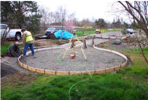
*Workers prepare the wooden form for the installation of a pervious concrete driveway at the Jefferson Nature Center Sports Park.*
