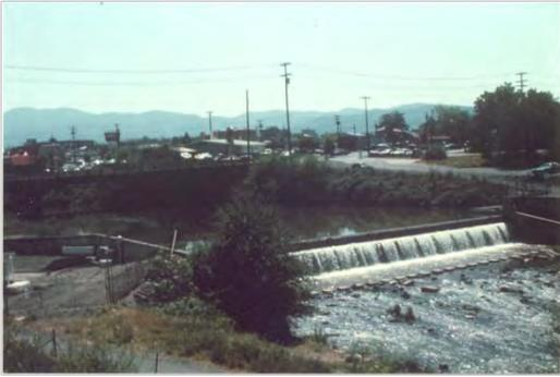
***Before:** An old concrete dam in Medford at Jackson Street disrupts the flow of Bear Creek making fish passage difficult. Lack of streamside vegetation allowed pollution to runoff into the creek.*
