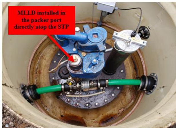
Figure 1.0 - Mechanical Line Leak Detector
