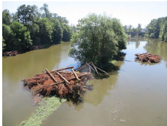
Engineered log structures in the lower Columbia Slough
