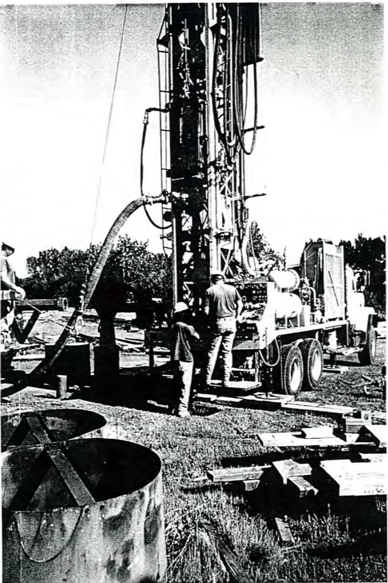
Drilling Monitoring Well MW-4
