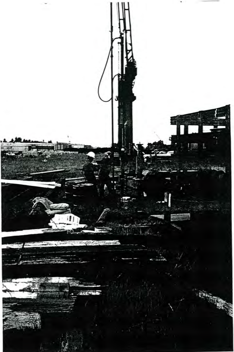
Drilling Monitoring Well MW-3
