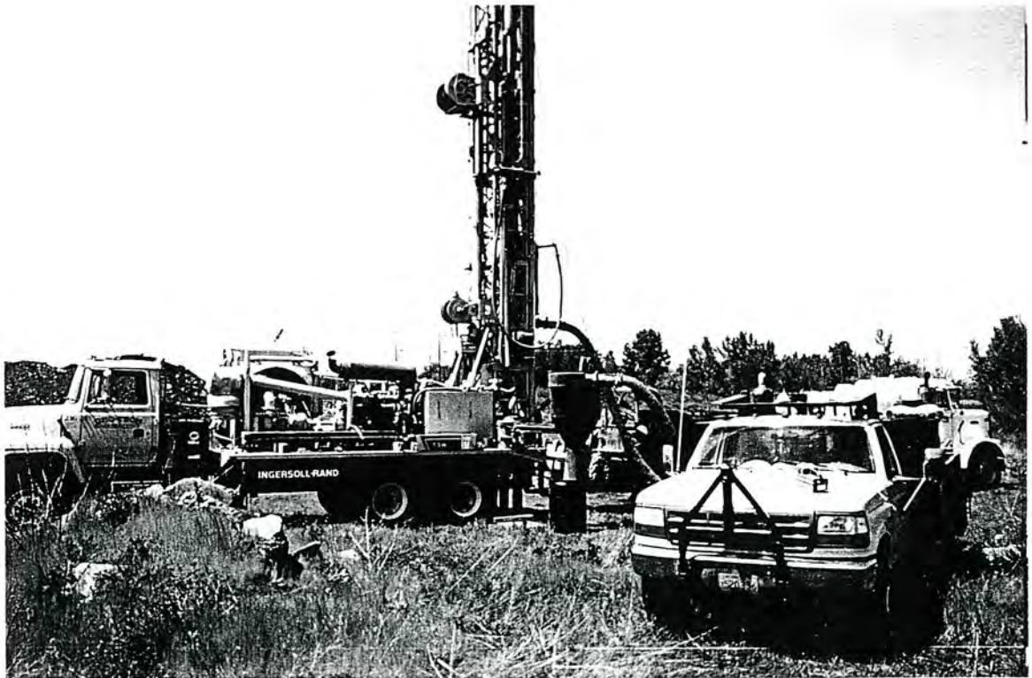
Drilling Monitoring Well MW-6
