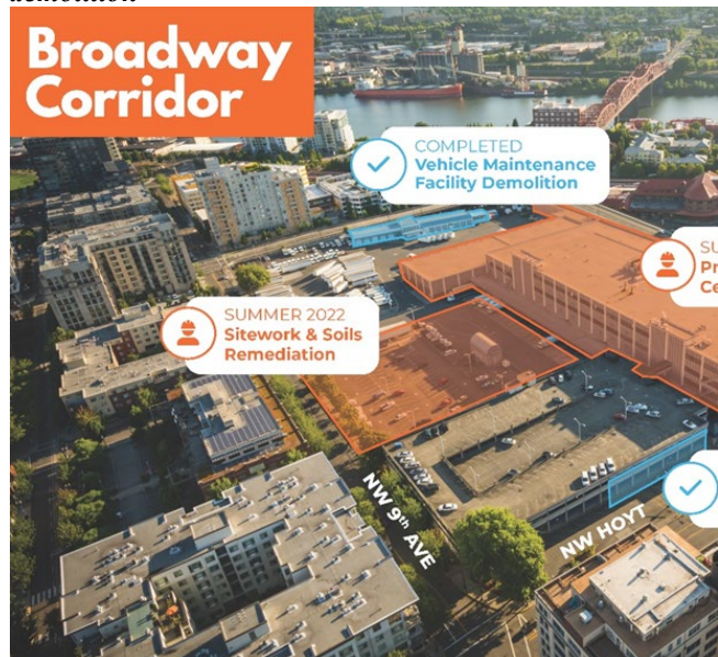
Figure. Prosper Portland's schedule for site work and demolition
