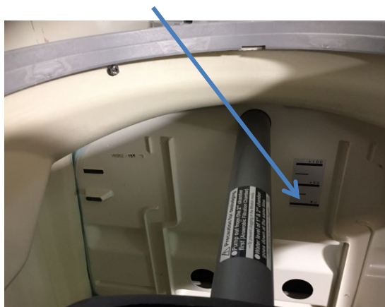
Low water line in sedimentation chamber
