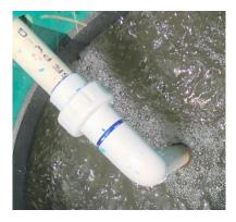
Splice "muffler" piece into the air line to help with noise from the aerator.
