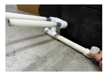
Glue vertical pipe to bracket and place in aeration chamber. Attached union and exit riser wall through grommet.
