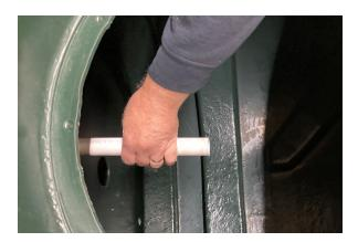
Cut pipe and glue second bracket piece.
