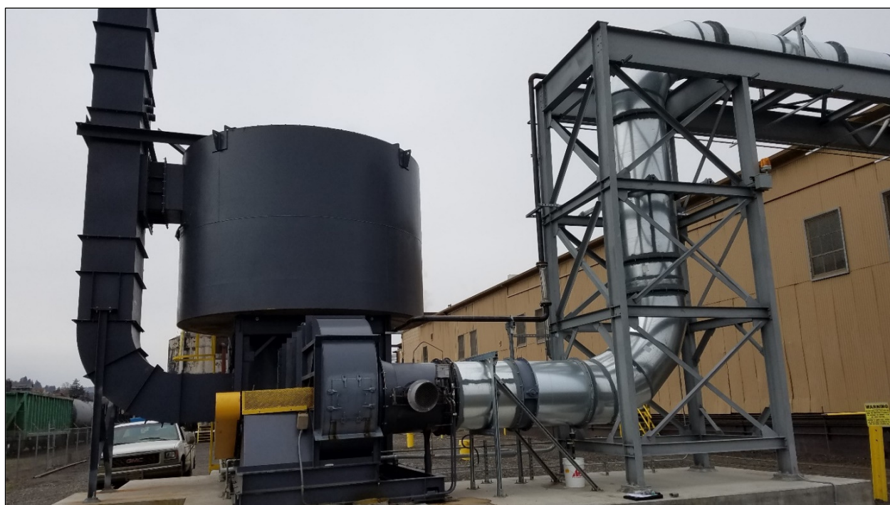
Figure 2: RTO Inlet Ductwork Photo.
