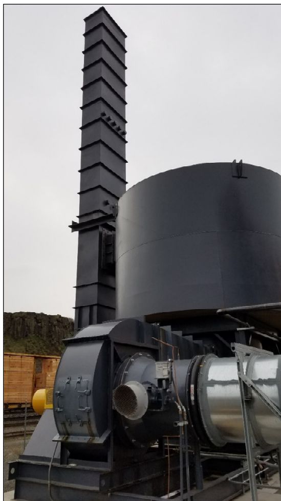
Figure 1: RTO Outlet Exhaust Stack and Sampling Ports.
