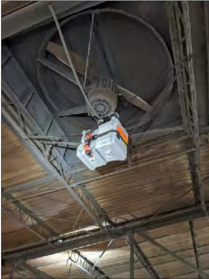
Figure 3. Building #11 Roof Vent 8
