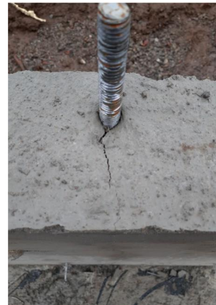
Photo 1 – cracking at foundation anchor bolt
