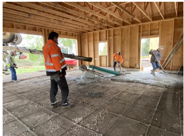
Photo 3 – pouring the garage slab
