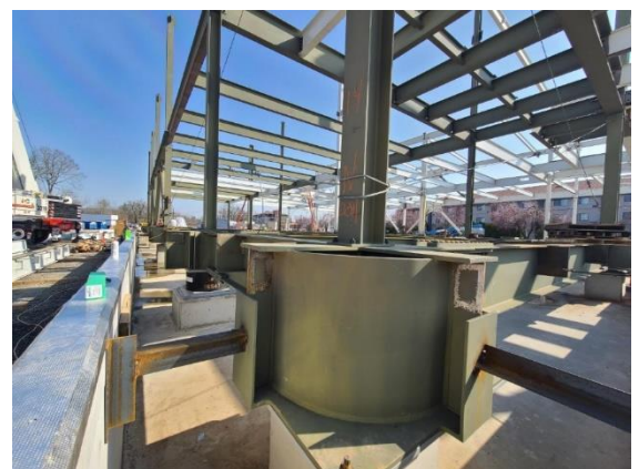
Base isolation node in the seismically stable foundation system
