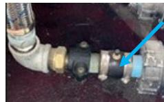
This STP sump sensor is correctly secured and rests in the correct part of the sump, flush with the bottom
