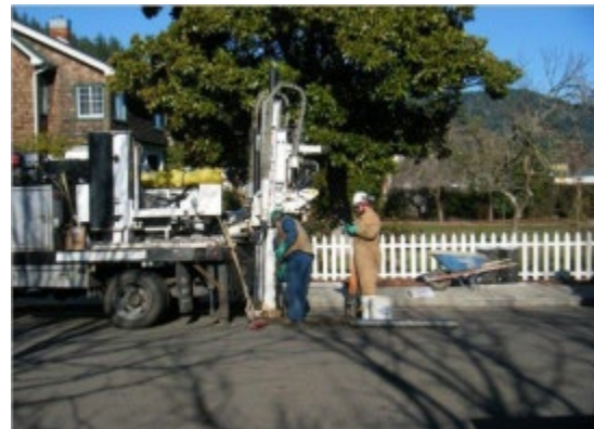
Collecting soil samples next to a leaking underground storage tank.
