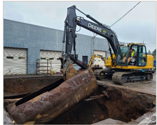
An environmental consultant removing an old steel underground storage tank.
