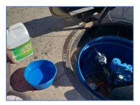
4) Slowly move the fuel float up until it triggers the high product alarm, and measure where that happens. Do the same with the water float. Check the measurements to make sure they correspond to the values programmed into the ATG.
