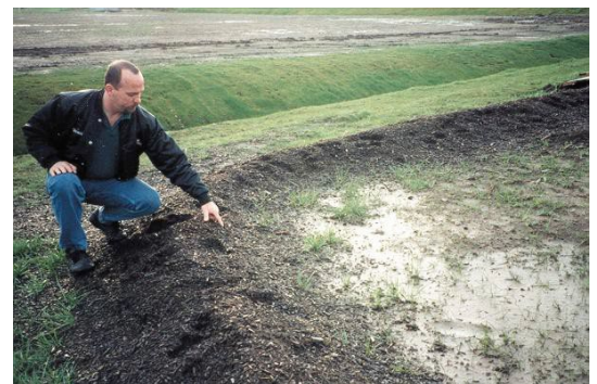
Compost berm to stabilize site.
