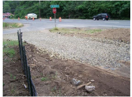
Gravelled site entrance.
