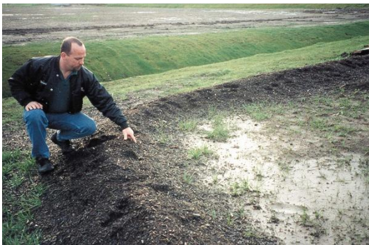
Compost berm to stabilize site.
