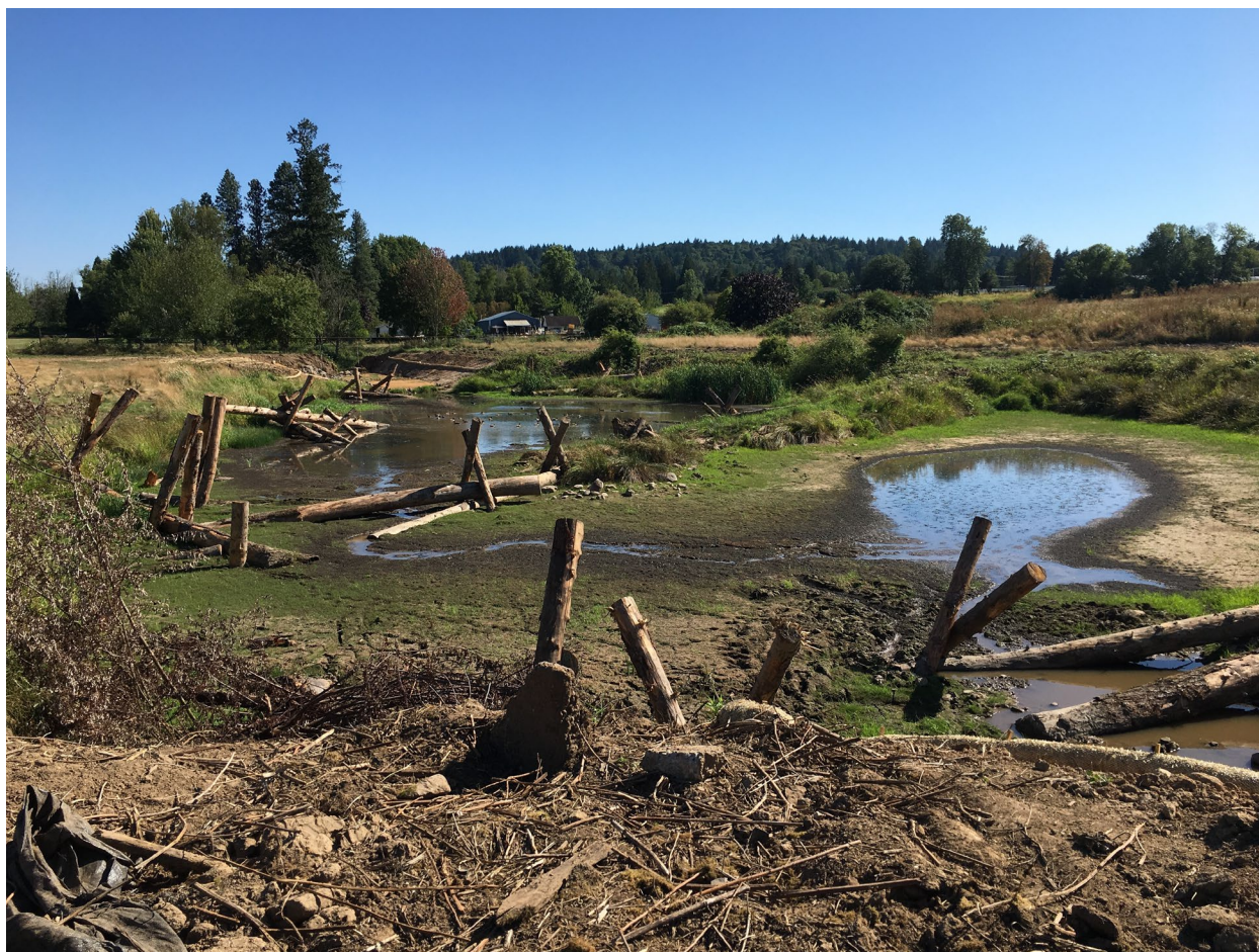
Figure R-2: Inline pond removed and fish passage restored on Mitchell Creek in the Johnson Creek watershed.
