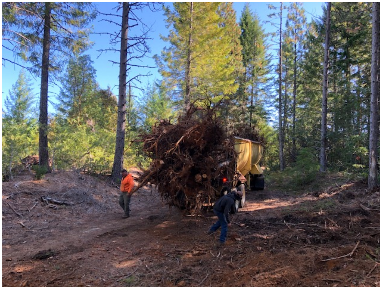
Figure M-3: Moving large wood for later instream placement. Photo Credit: Kevin O'Brien, Illinois Valley Watershed Council.
