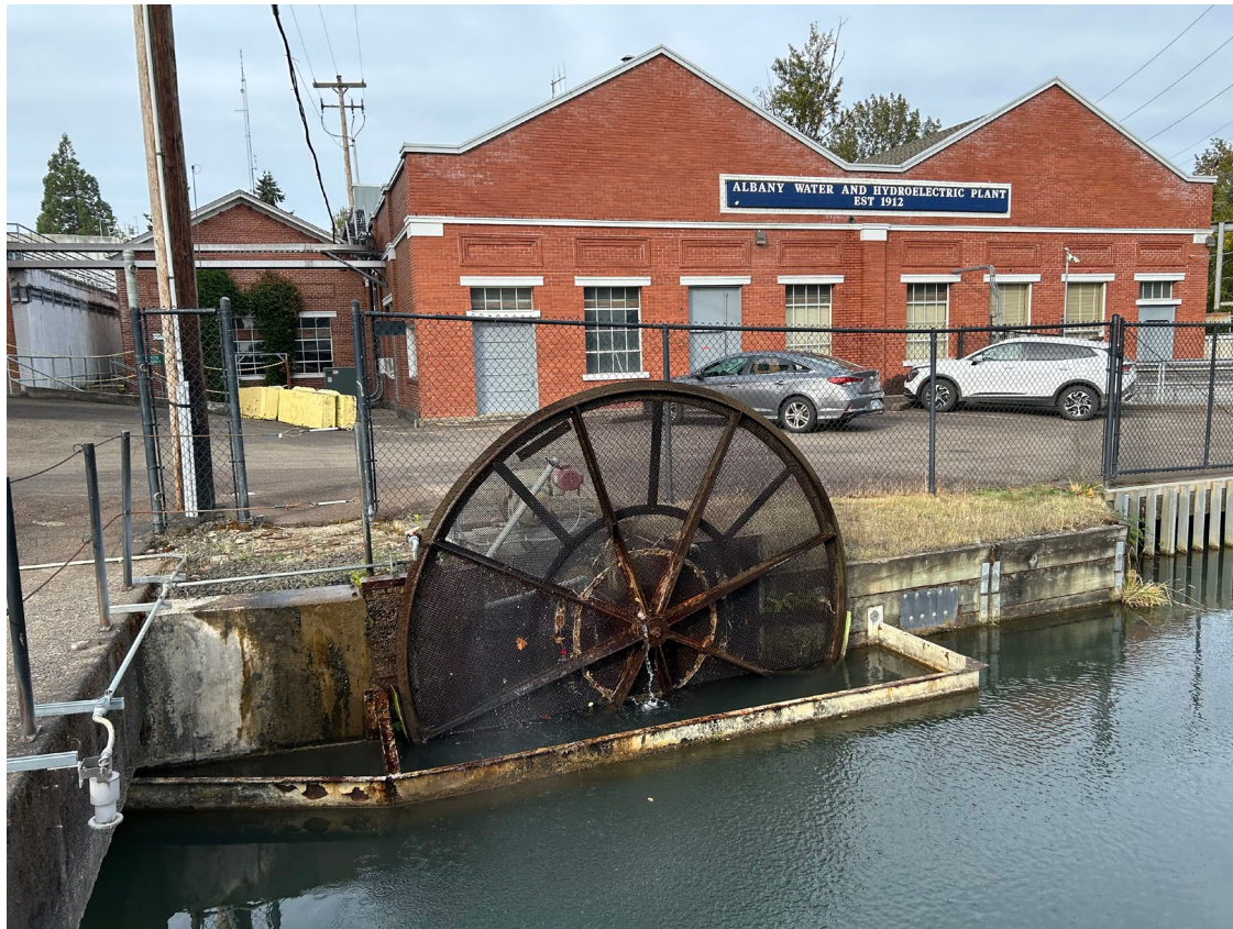
Photo Caption: The drinking water diversion occurs at the point of the round, wheel-shaped screen in the middle of the photo. The hydropower water diversion occurs at the point of the vertical barred screen on the right side of the photo.
