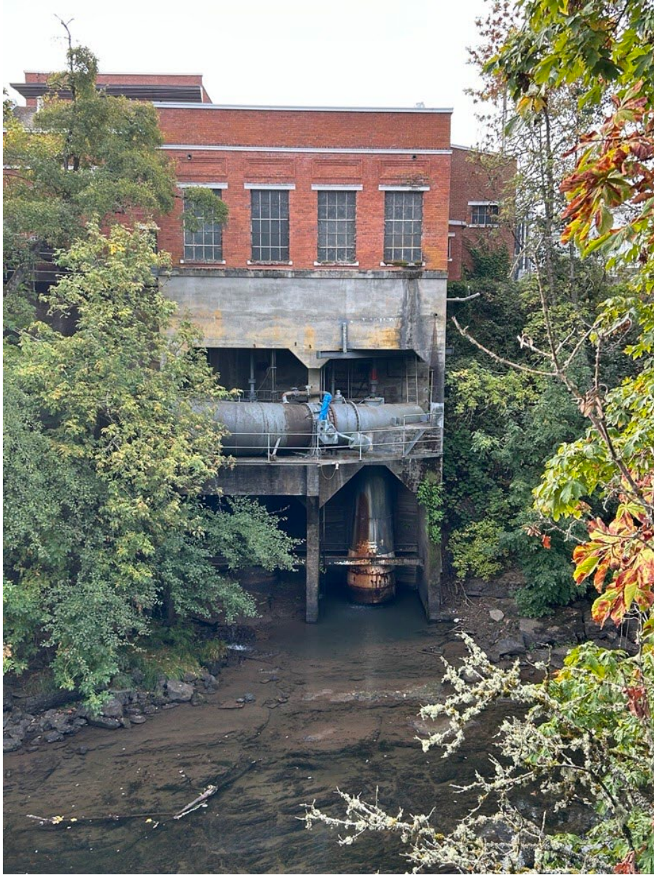
Photo Caption: Albany Hydroelectric Project draft tube point of discharge into the Calapooia River. Project is shown during non-operational condition. October 2025.
