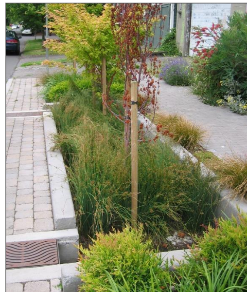
Bio-swales collect stormwater runoff from roadways and then slowly filter it through layers of soil, sand and stone.
