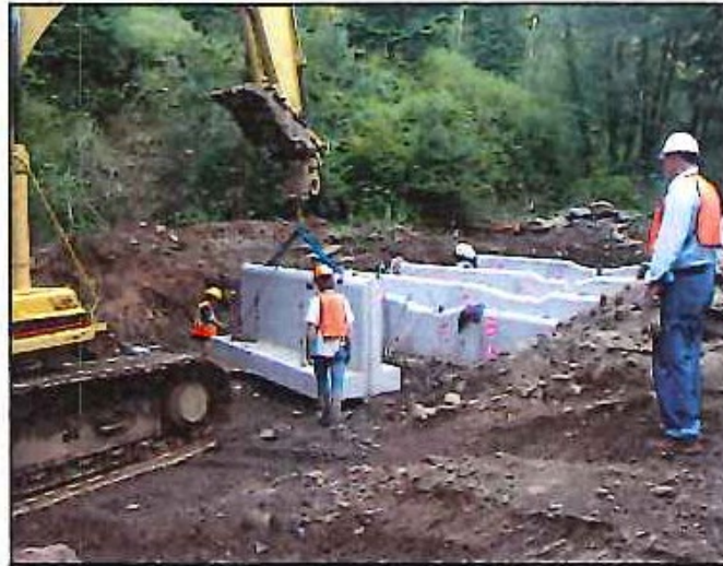
Sept 22, 2009: During Construction
