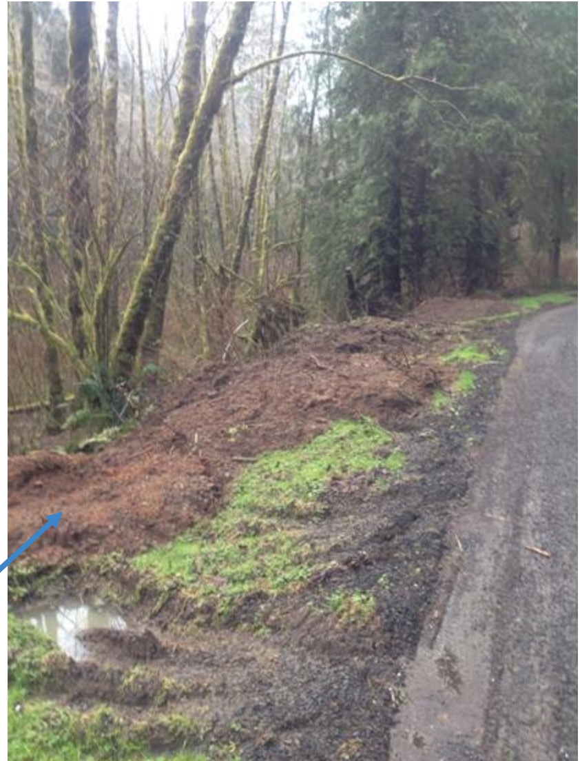
Sidecast soil from road maintenance
