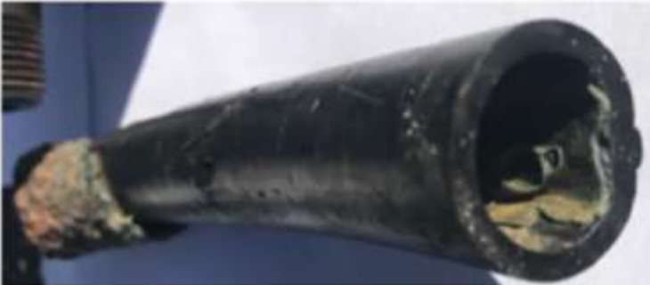
Whole view of pipe A with A melted plastic inside (A1) and melted plastic on outside (A2)
