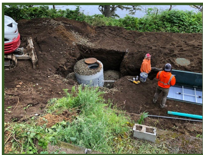
An approved alternate treatment septic system is installed near a waterway in Tillamook County
