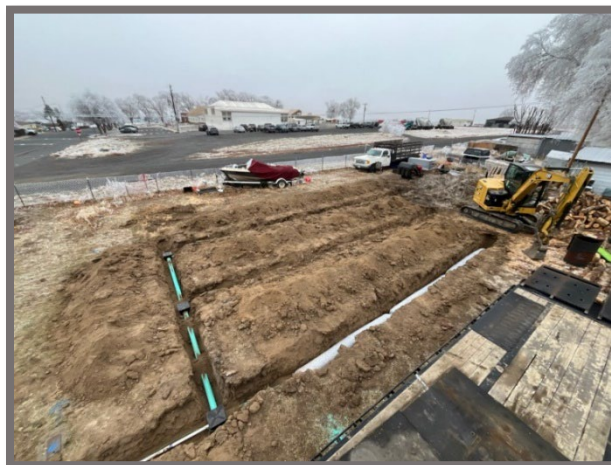
A drain field is installed as part of a major repair in Deschutes County.
