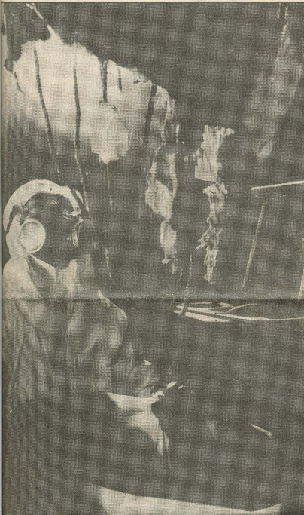
Abatement worker strips asbestos insulation from air duct.
