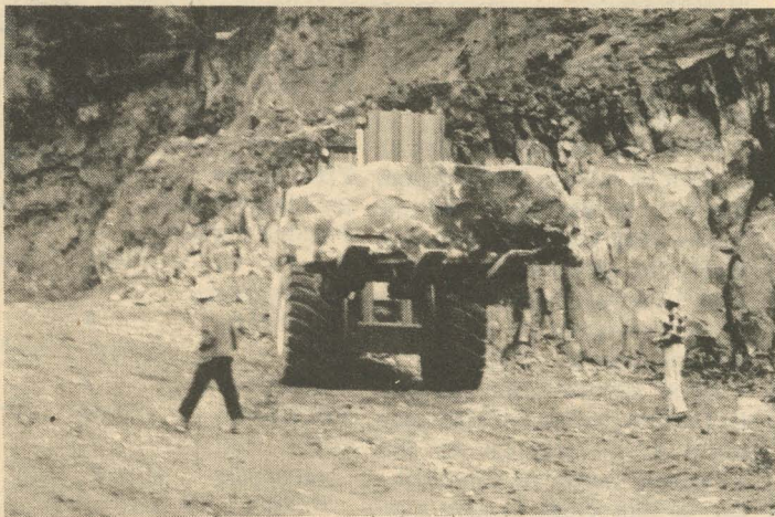
THIS GIANT ROCKHOUND is ready to load onto an Asbury truck. Action took place at the huge quarry near Siletz where rock is being gathered for the North Jetty at Newport. (See additional pictures in this week's News, Page 1, Section 2.)
