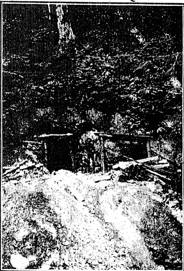
SHOWING TUNNEL MOUTH AT THE BLOOMFIELD.
