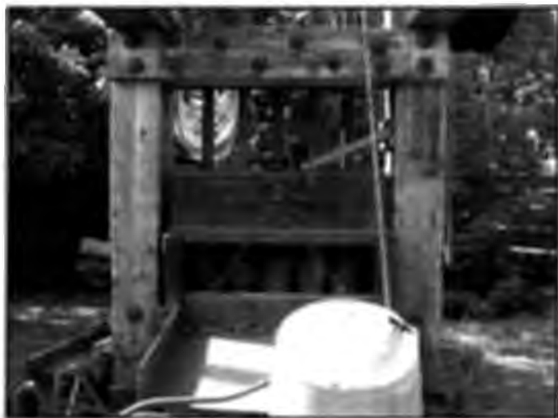
View of the lower portion of the stamp battery. Note the stamp heads.
