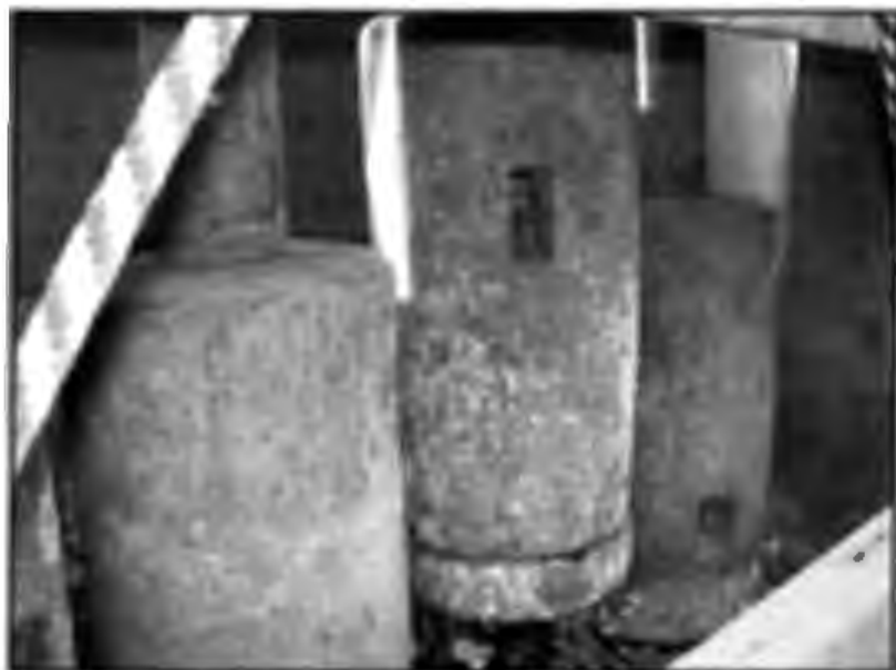
View of the lower portion of the stamp battery. Note the stamp heads.
