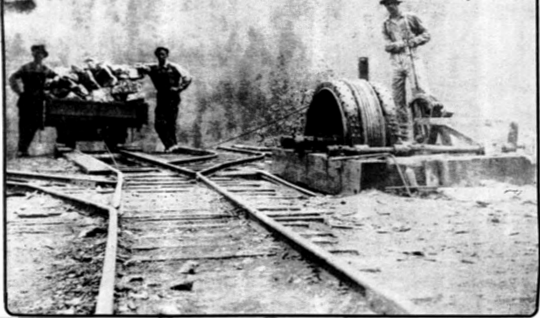
Tram & hoist at the Lively Lime quarry on Kanes creek around 1930. Steam engine, not in photo operated the works. Note wooden blocks on the friction bands used as brake & clutch. Men in photo not identified. This was a large industry in Gold Hill for many years. courtesy Winona (Shoemaker) Nichols
