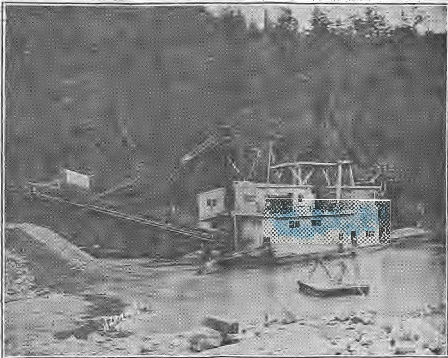
The Eddiam gold dredge, which was assembled during 1925, has been operating recently in the Foots-Creek district. The big dredge floats in a small lake and pulls from the bank, guided in operation from side to side. Water for the lake comes from the creek and its position is changed as the big machine progresses. A great steel pipe under the supervision of E. H. Perry, keeps the dredge busy, day and night and it is estimated, there is an area of operation sufficient to keep the machine in operation for at least 10 years at the present rate.
