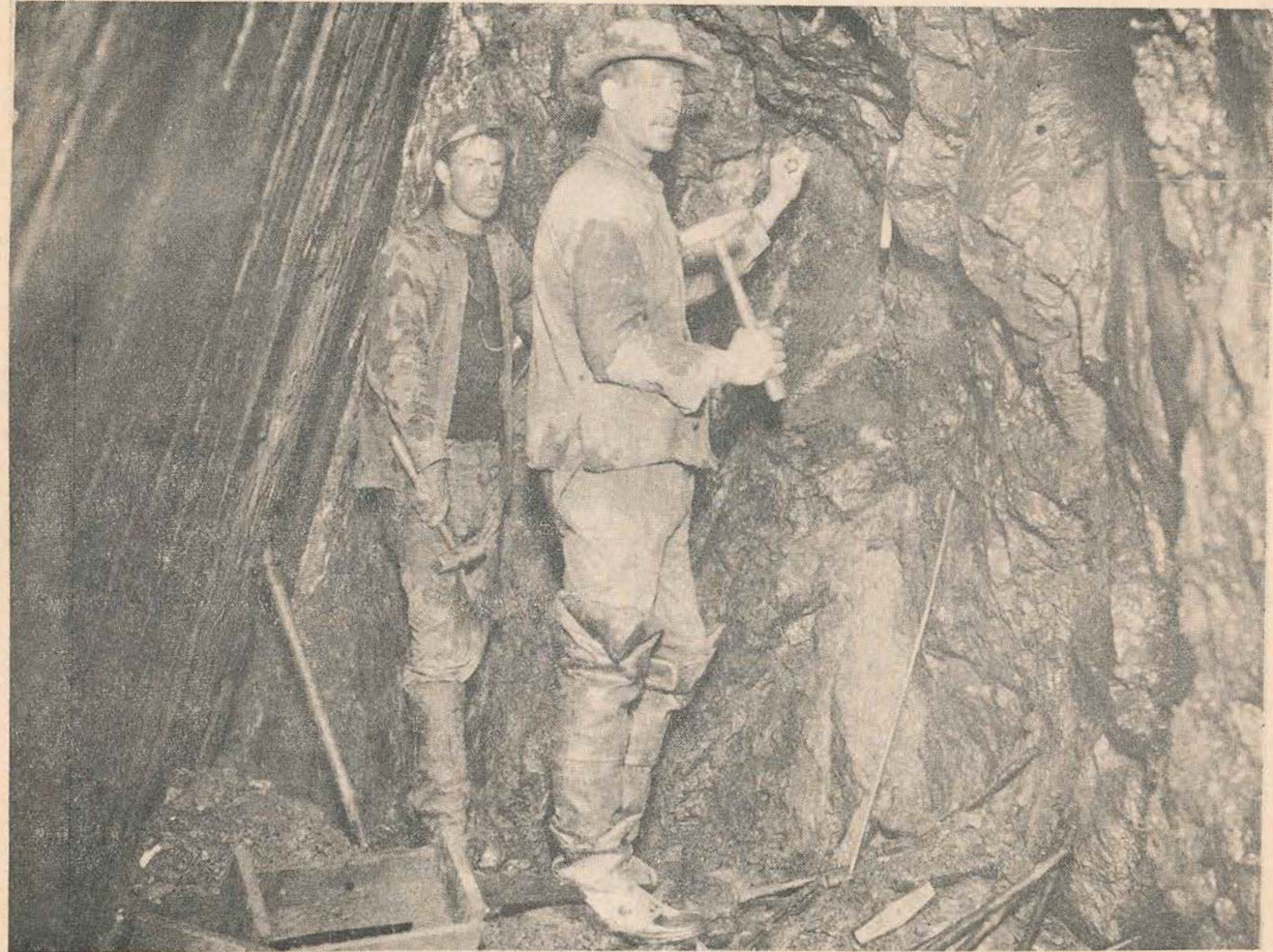
SINGLE-JACK MINERS — These two miners, Hugh Grant and Charles McCormick, were snapped while at work on the second level of the Golden King Mine, near Alleghany, Sierra County, California, in May, 1894. "Single-jacking" is largely a forgotten art, as machine drills have replaced this method of making
