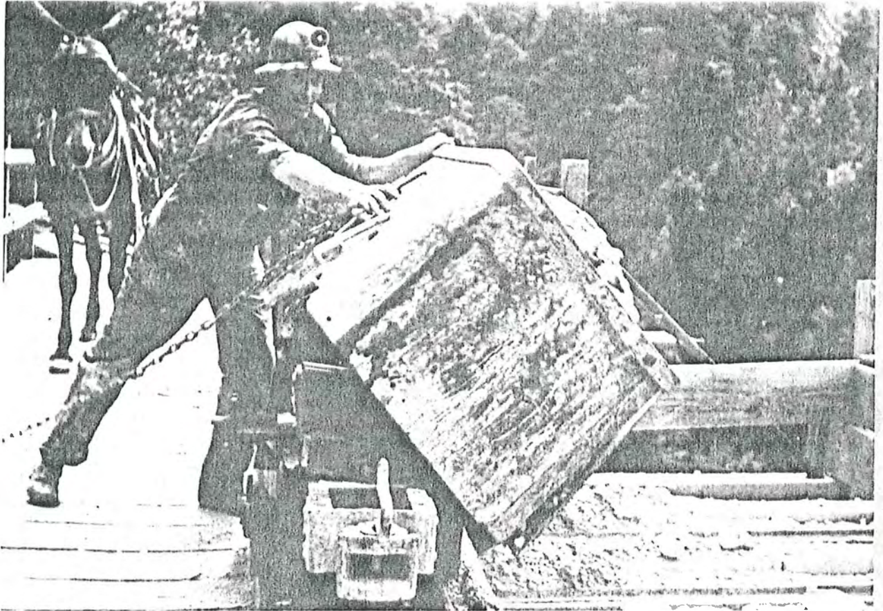
Unloading an Ore Car
