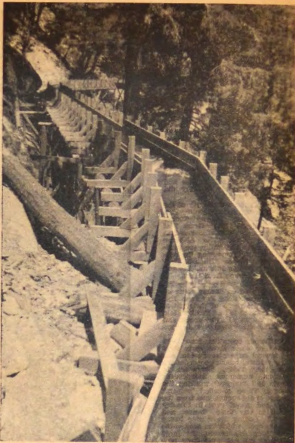
View of newly constructed flume at Gold Bond Placer, carrying water from the creek to be used in hydraulicking. The rugged country at this point gives the water considerable "fall."
