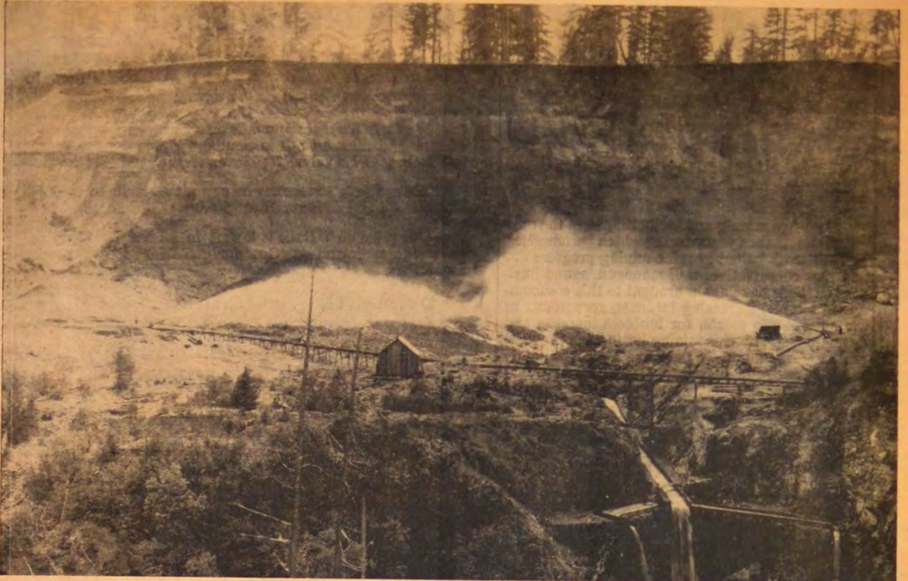
Showing operations at the Old Channel mine, with two "giants" trained on the base of the gravel bank. This breaks down the bank by undermining it below, allowing the material to wash into the sluice which may be seen in the right foreground. The "fines" are caught by the riffles and the coarse material passes on and down the fall. The elevated pipe line carrying the water to the "giants" may also be seen.
