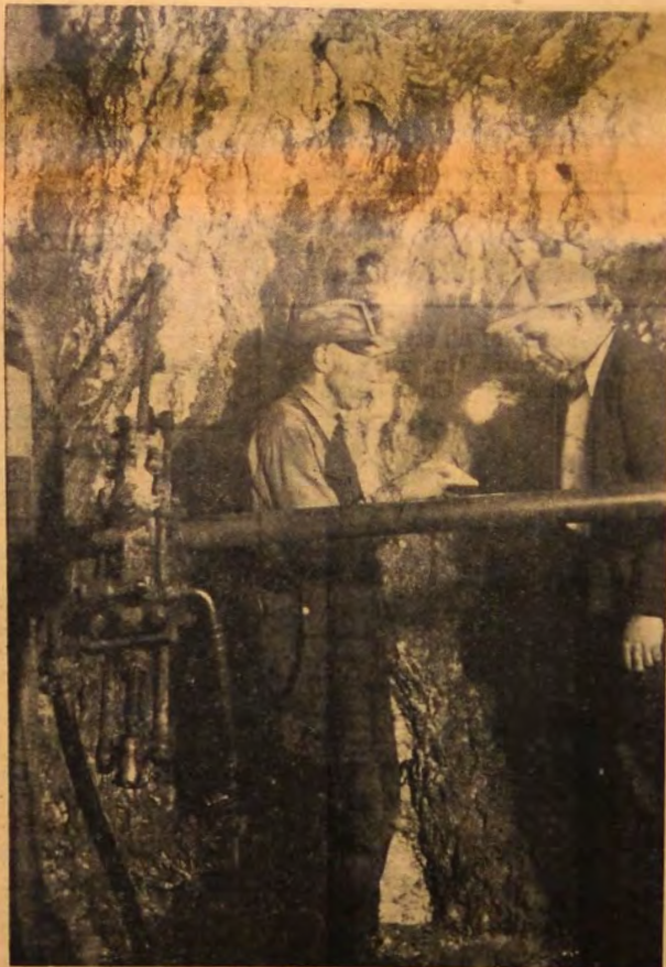
Miners with air drill one of the tunnels at the Oriole mine, one of the important quartz properties in the Galice district. The mine is owned by Harry Sordy and is being operated under a lease by Charles Benson and Ben Thomas. Several thousand dollars have been spent during the past year in new equipment.
