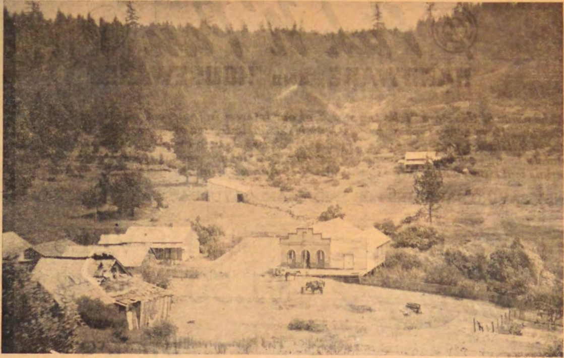
Old townsite of Waldo, which is being gradually torn away by the giants of the nearby placer mines, except the site where the store built by A. B. McIlwain in 1863, still stands in a state of decay.
