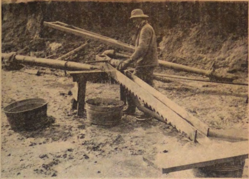
Re-washing concentrates in sluice box at Esterly mine during past year's operation on Nixon property. Operating crews ready to start again as soon as weather and water permit.
