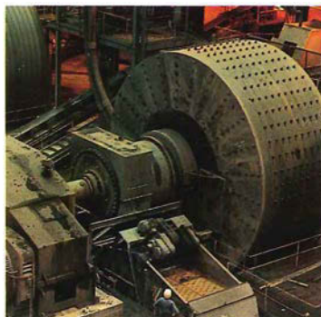
Huge mills, left, grind iron-bearing rock into fine grains so the particles richest in iron can be freed and rolled into pellets containing 60-65 percent iron.
