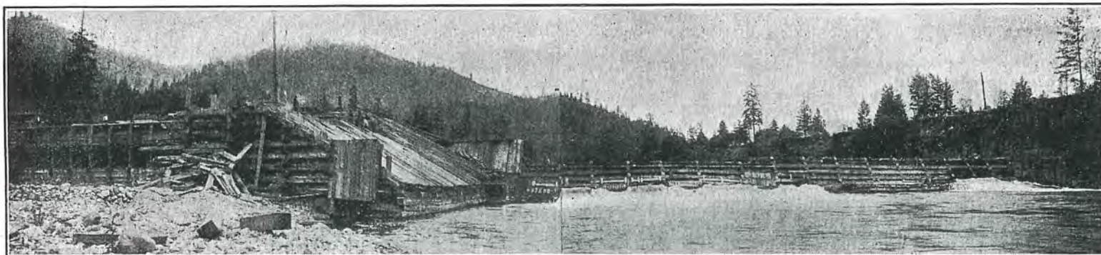
DAM OF GOLDEN DRIFT MINING COMPANY, ACROSS ROGUE RIVER, FOUR MILES ABOVE GRANTS PASS.
