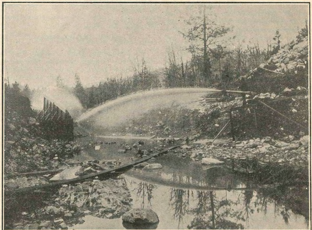
SHOWING A RUBLE GRIZZLY AT WORK. THE SCAFFOLD SUPPORTING THE GIANT IS NOT A NECESSARY PART OF THE APPARATUS.
