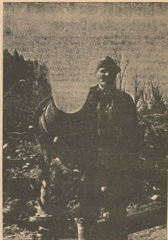
NUGGET'S EYE view of Harry Steward guiding a powerful jet of water toward paydirt. The thundering stream of water will blast loose gold-bearing gravel and wash it to the sluices, where the gold is separated from the dirt and gravel, becoming trapped in the riffles. Steward is one of Josephine County's long time miners, and active in the Sourdoughs.
