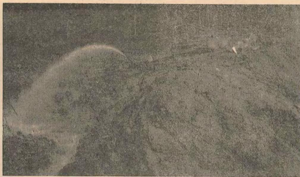
LET WATER do the work. A thundering jet of water tearing loose gold bearing gravel and washing it through a sluice is the most economical method of mining. Placering is usually done in winter when water is available and the miner must work out in the inclement weather to get that magic metal, gold.
