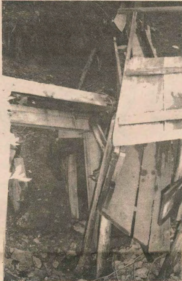
CAVED-IN TUNNEL off Waldo Gulch.
