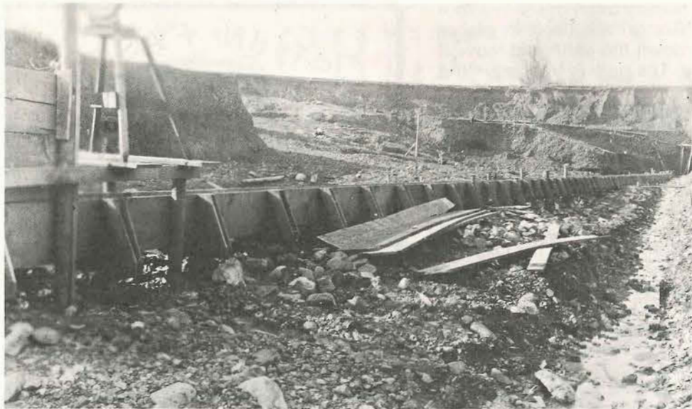
The flume "that catches the gold" in the lower pit of the Logan Mine near Waldo, OR.
