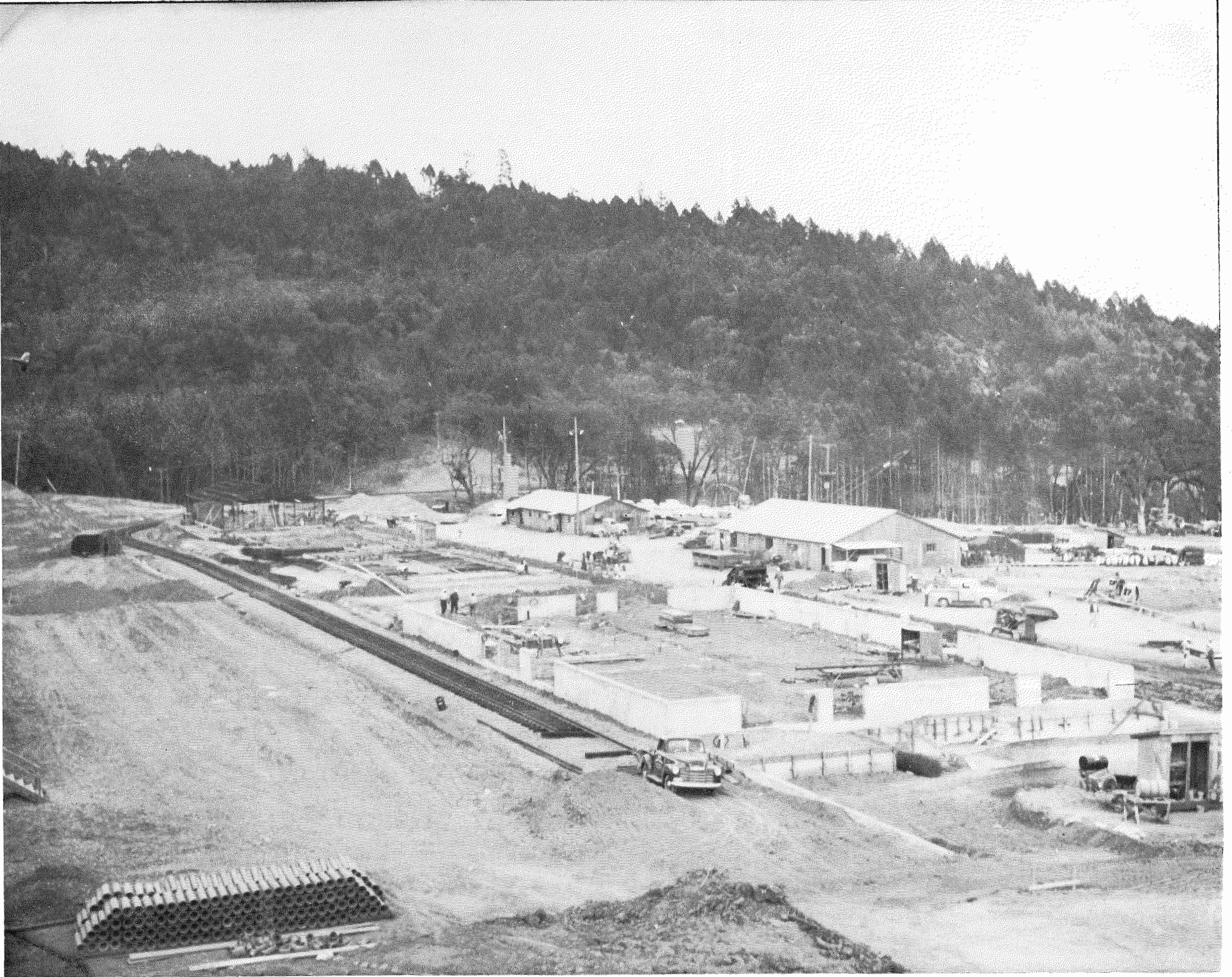
FOUNDATIONS FOR STORAGE LABORATORY AND OFFICE BUILDINGS. RAILROAD SIDING IS SHOWN. ; FOUNDATIONS FOR MAIN ELECTRIC FURNACE NICKEL SMELTER
